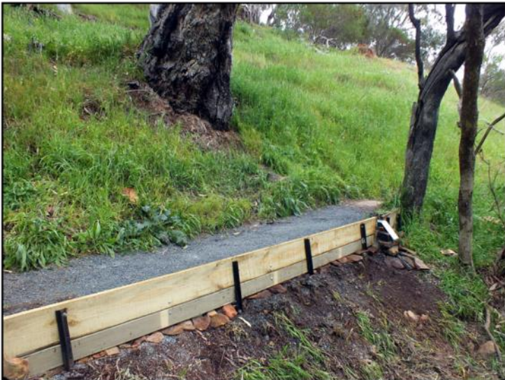
Reconstructed section in Netherby Gully
