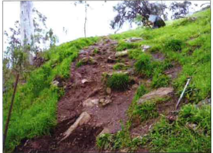
Walking trail damage
